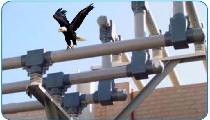
Joint Insulation at a Power Substation
