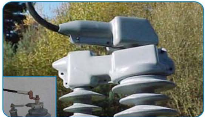
Terminal connection on the Recloser
