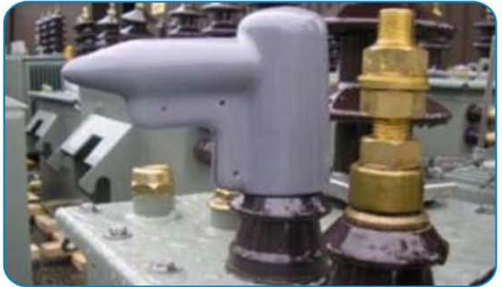
Terminal and Cable Lug on the VT bushing
